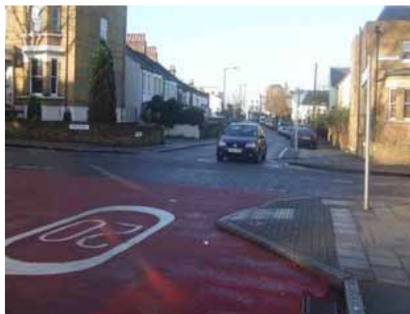
Figure 4.4 Coloured surfacing at zone entry
